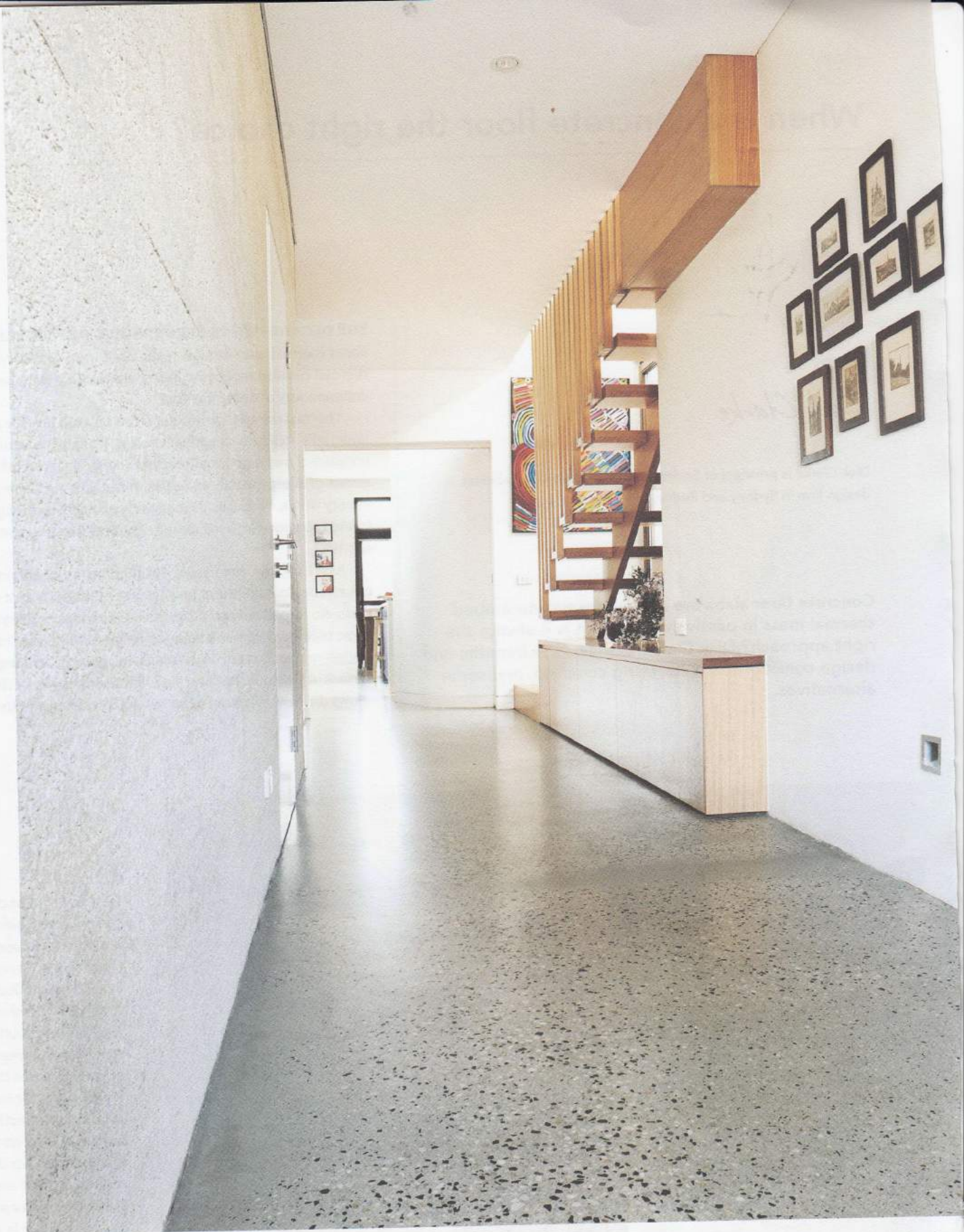
① This Melbourne home's polished concrete floor includes 30 per cent flyash with a lovely aggregate pattern exposed in polishing. The slab edge is insulated with R1.5 Foilboard and the floor is finished with Kunos Natural Oil by Livos. Image: Rhiannon Slatter. There is a profile of this Steffen Welsch Architects design in Sanctuary issue 25.
