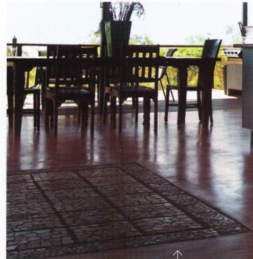
Concrete thermal mass in the shaded floor cools the interior and adds a striking visual component
