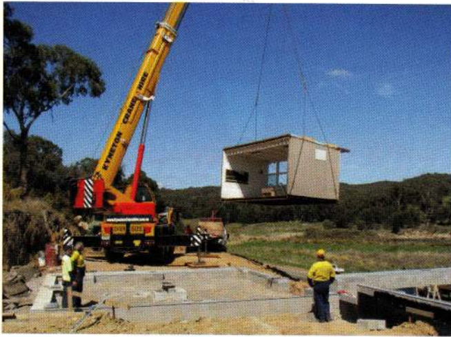
↑ Half a portable being craned into position (above), and the two portables installed (right).
