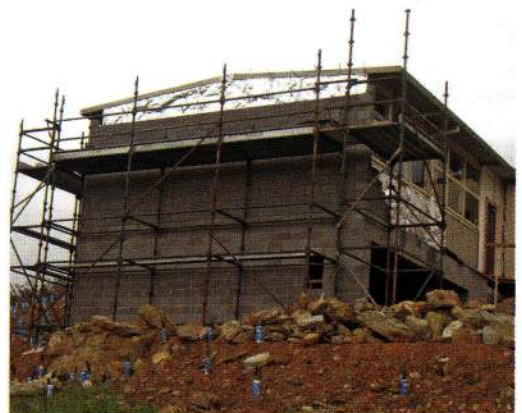
↑ The blockwork going on one of the portables, with foil insulation underneath.
