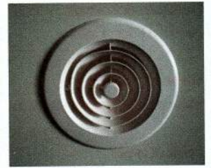
↑ This wall mounted interior grille is installed in the upper rooms. When turned on it transfers heat through ducts to the cooler rooms of the home. Photo by Verity Campbell
