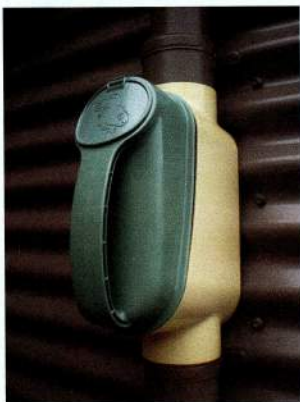
↑ The Tadpole downpipe filter is fixed at shoulder height and is easily removed for cleaning. Photo by Verity Campbell
