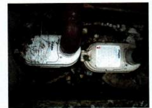
↑ Shown here are both Nylex Greywater Diverta units for the home. Photo by Verity Campbell
