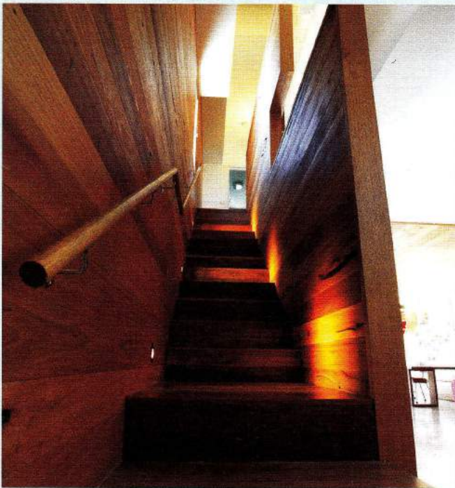
① Positioned above the striking recycled timber staircase, a small operable skylight brings in light and vents heat.
